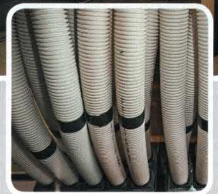
Tubes deliver heat and exchange air from the heat pump to the whole house
